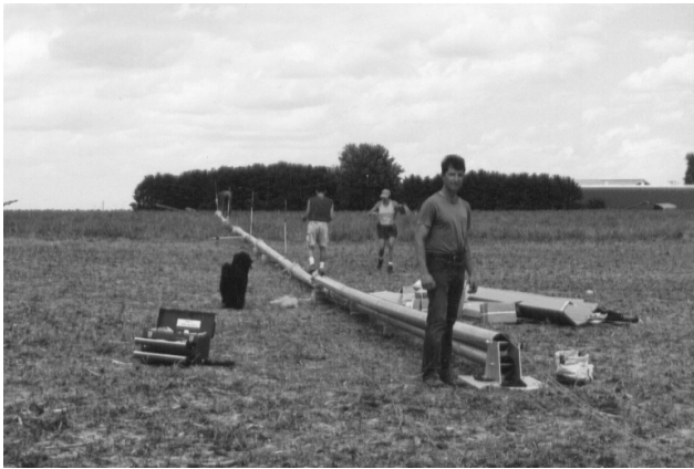
Erecting Test Tower – Lake City
