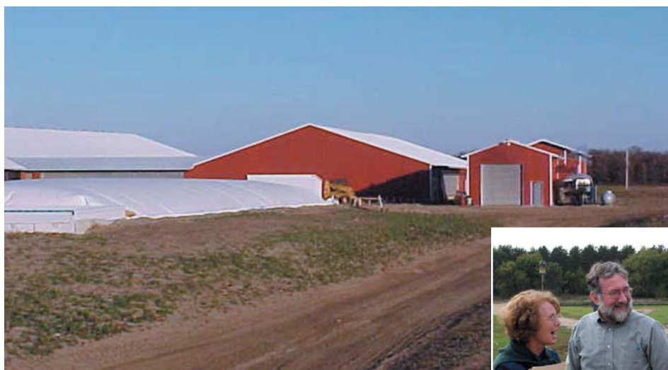
Haubenschild digester barn and electrical generation building is shown above. Dennis Haubenschild (right) visits with field day tour participants.
