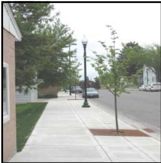
Norwood main street improvements
