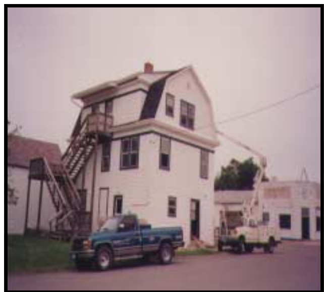
Renovation on historic hospital
