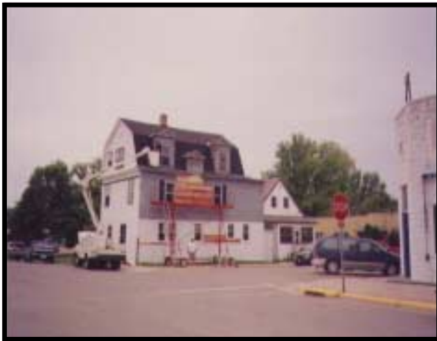
Hospital renovation in progress
